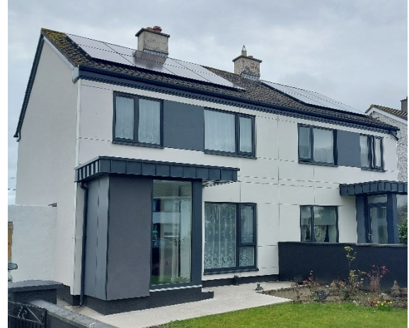
Before and After: Circular renovation pilot in Athlone
